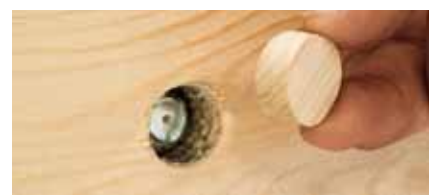
7. Cover hole with end-grained wooden plug.
